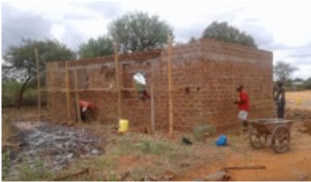
Work in progress...the New Church near Voi. Roof needed-$3000
